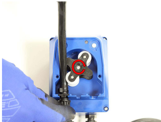
Fig. 71 Position the roller at 7h01
