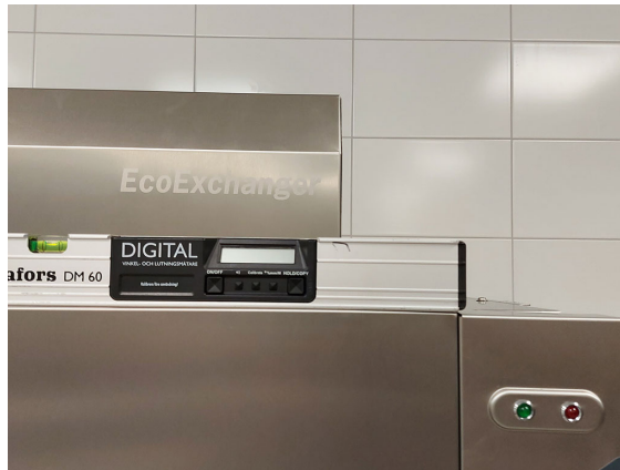
Fig. 3 Leveling front.
